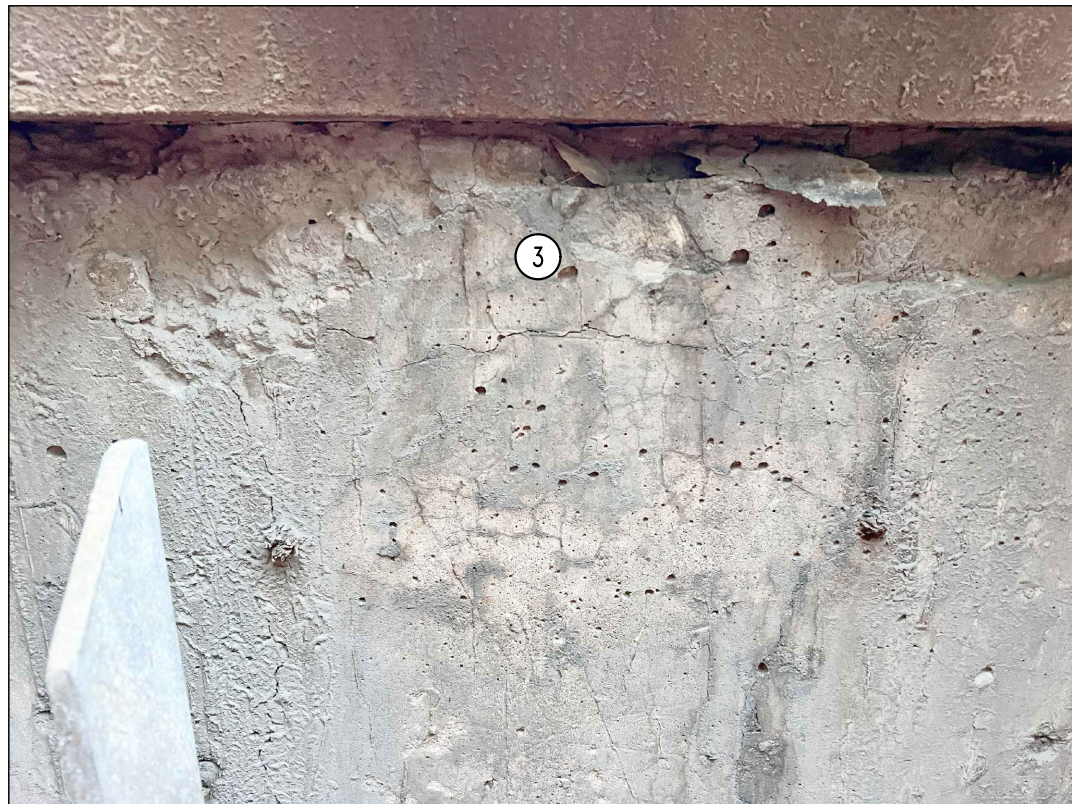
3 SPALLING UNDER MANHOLE LID. SEE NOTE #3.
