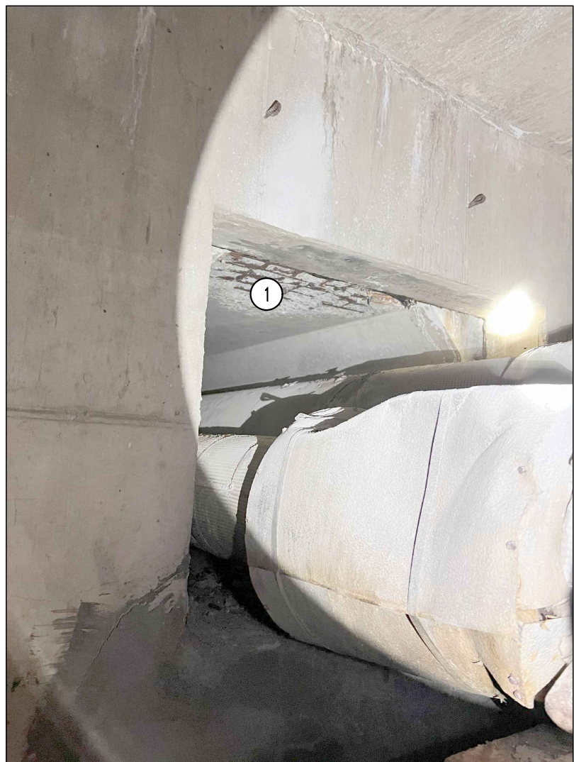
1 REBAR EXPOSED, WEST CHASE LID. SEE NOTE #1.
