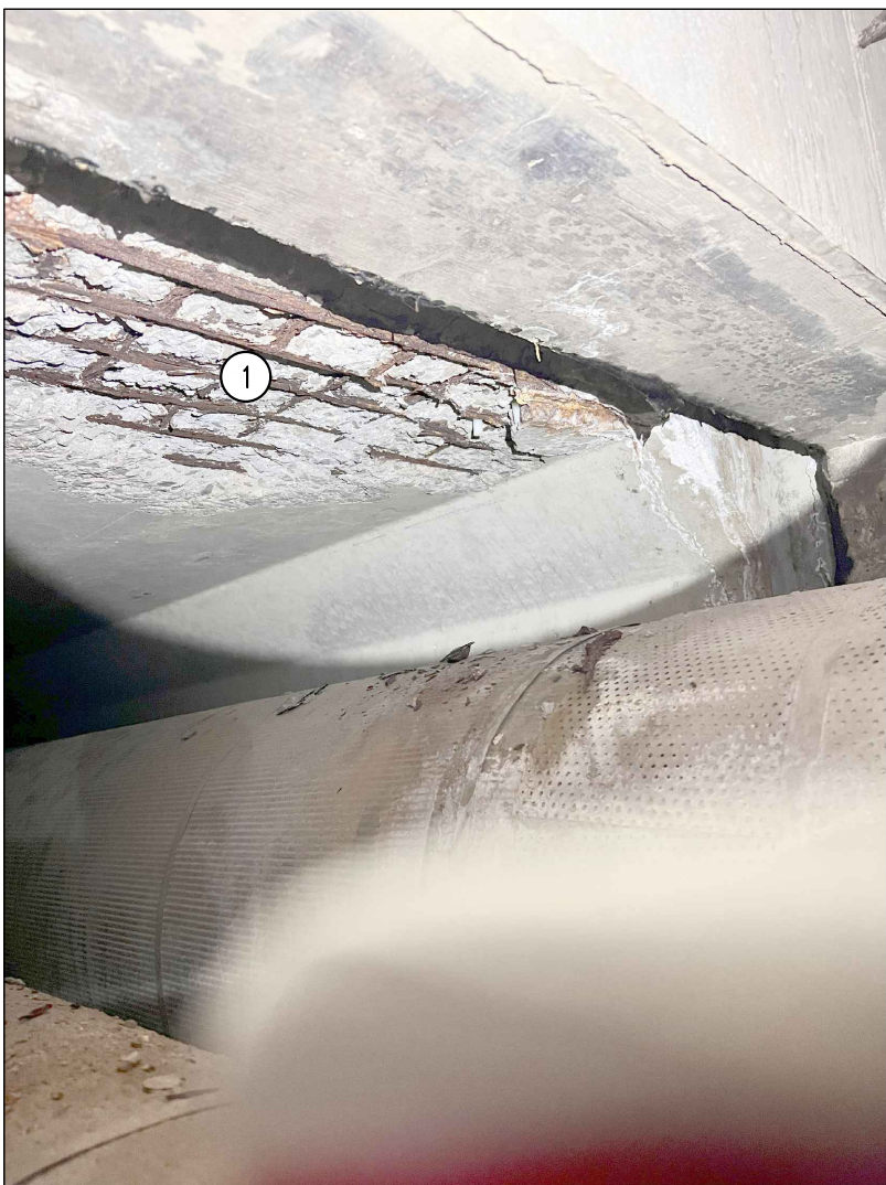
1 REBAR EXPOSED, WEST CHASE LID. SEE NOTE #1.
