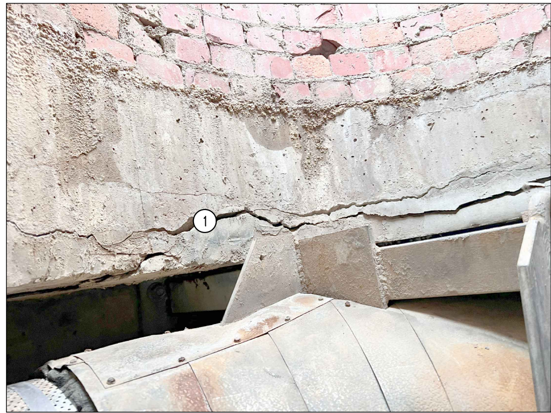
1 LID CONCRETE SPALLING. SEE NOTE #1.
