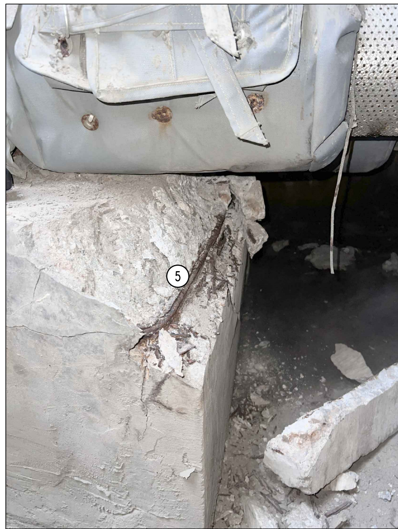
5 EAST CONCRETE ANCHOR SPALLING. SEE NOTE #5. NOTE: STEAM LINE WILL REMAIN ACTIVE.
