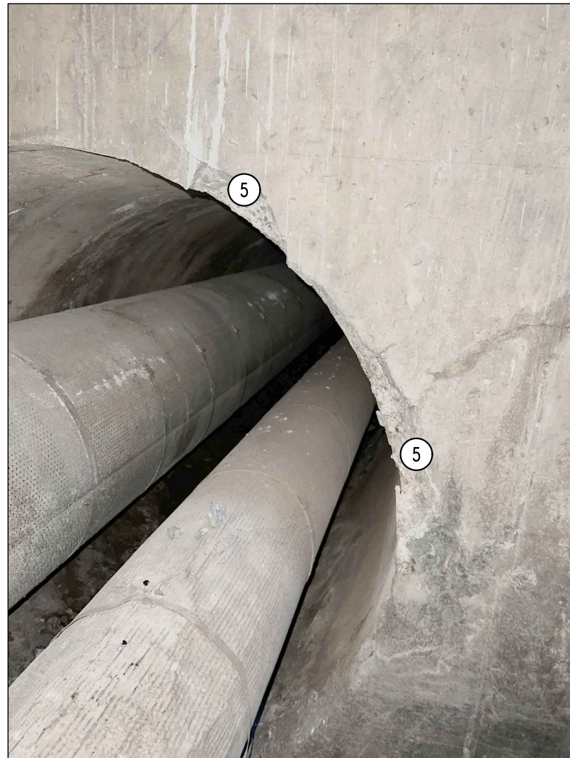
5 EAST CHASE SPALLING. SEE NOTE #5.
