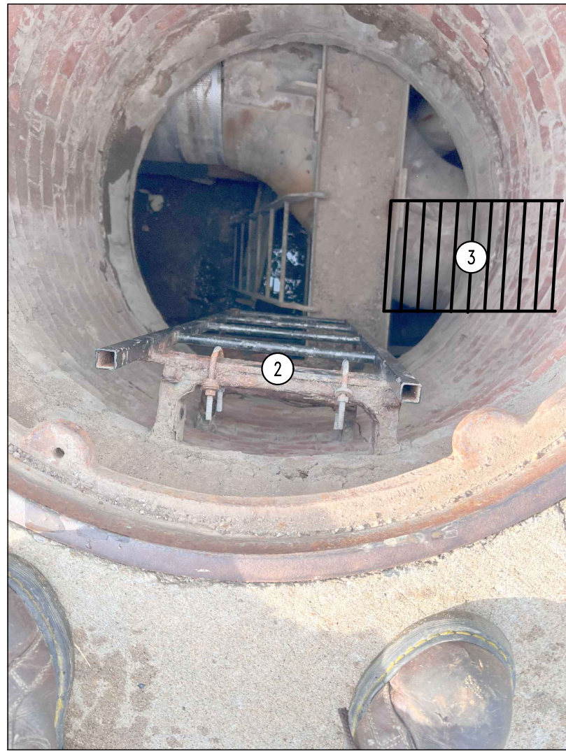
2 REMOVE EXISTING LADDER @ NORTH SIDE. 3 NEW 20" WIDE x 66" TALL GALVANIZED LADDER w/ #6 REBAR RUNGS INSTALLED ON WEST SIDE OF MANHOLE. PROVIDE 1/2" BENT PLATE & 1/2"Ø GALVANIZED A307 THREADED ROD w/ 4" HILTI HY-270 EPOXY EMBEDMENT. TOTAL (4) ANCHORS (FIELD VERIFY DIMENSIONS PRIOR TO FABRICATION).
