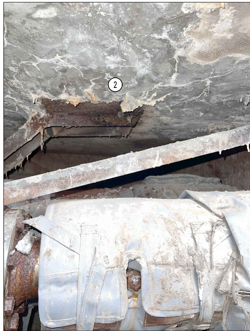
2 WIDESPREAD LID SPALLING. SEE NOTE #2.
