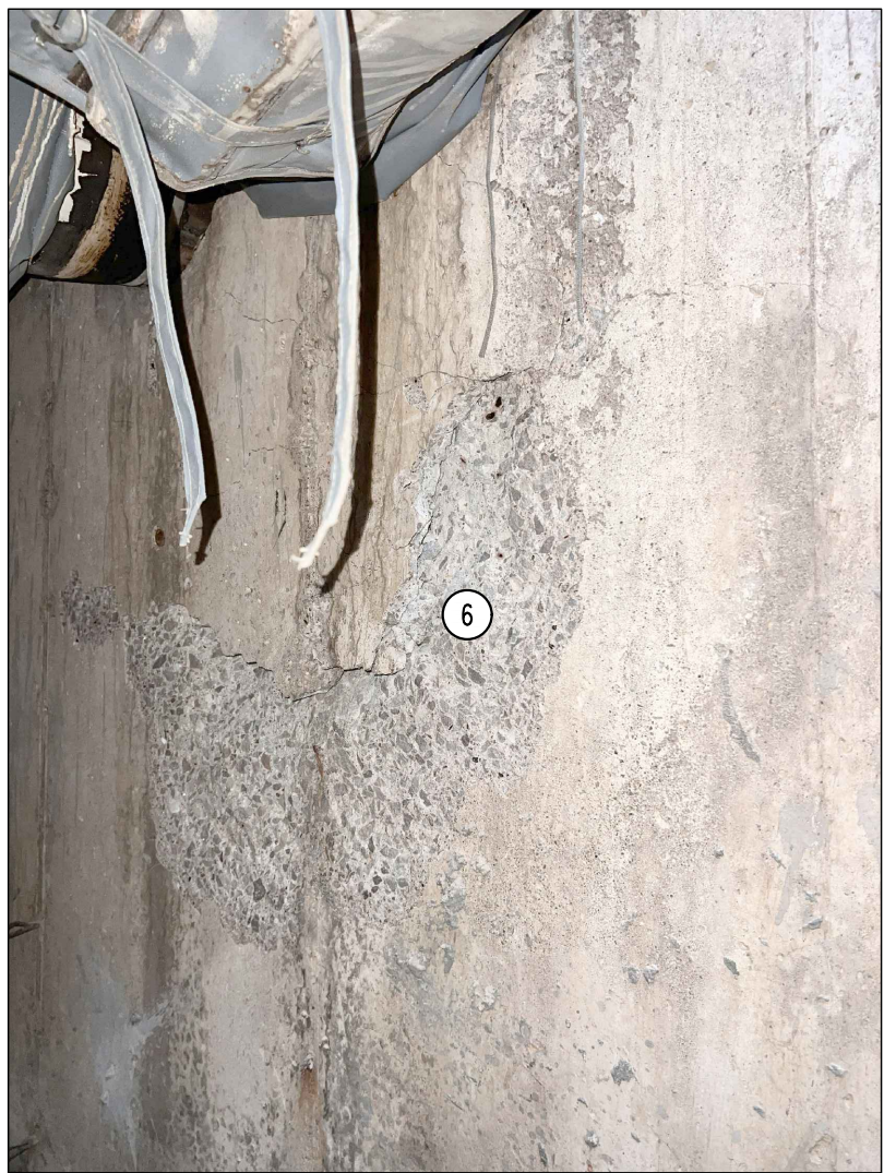
6 NORTH WALL CONCRETE SPALLING UNDER PIPE. SEE NOTE #6.
