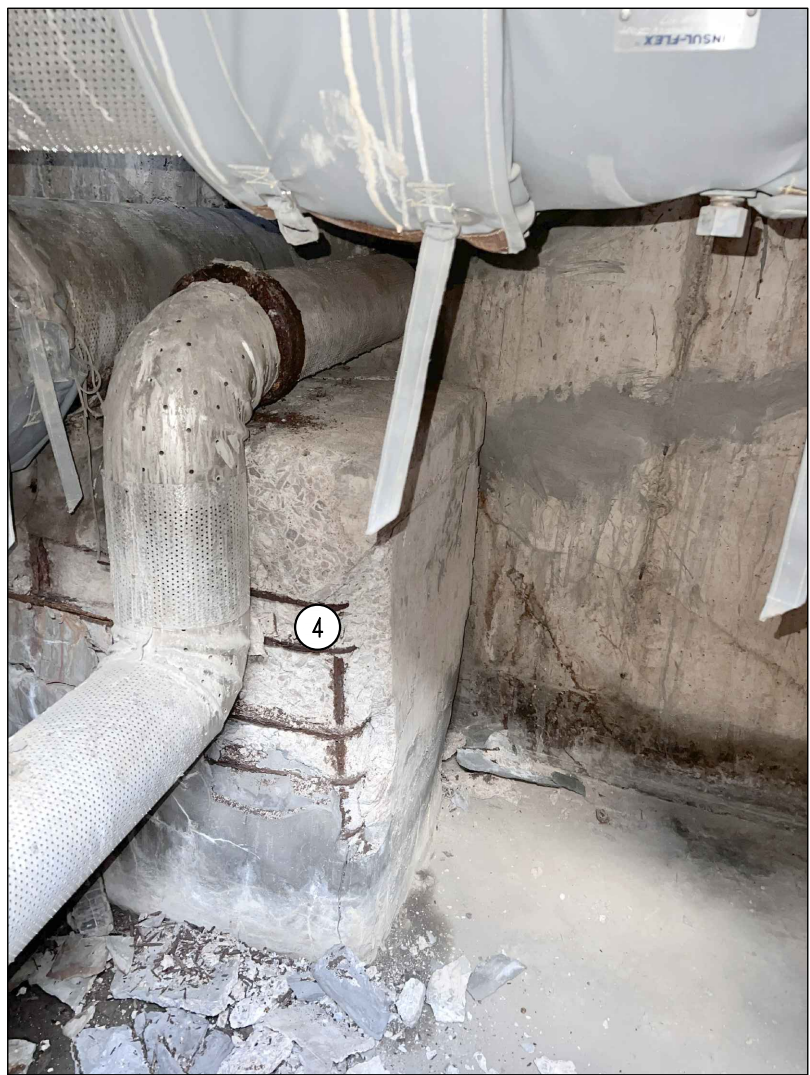
4 WEST CONCRETE ANCHOR SPALLING. SEE NOTE #4. NOTE: STEAM LINE WILL REMAIN ACTIVE.
