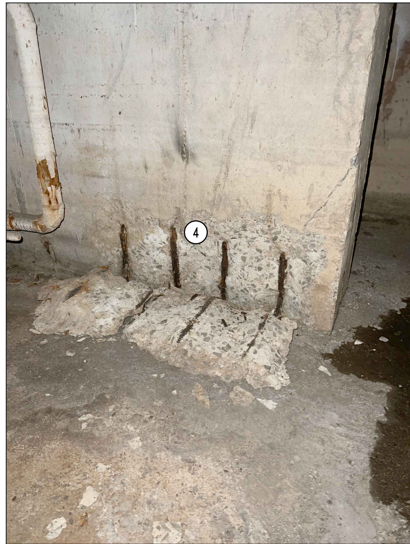
4 CONCRETE SPALLING WEST SIDE OF NORTH/SOUTH ANCHOR WALL @ SOUTH END, SEE NOTE #3.
