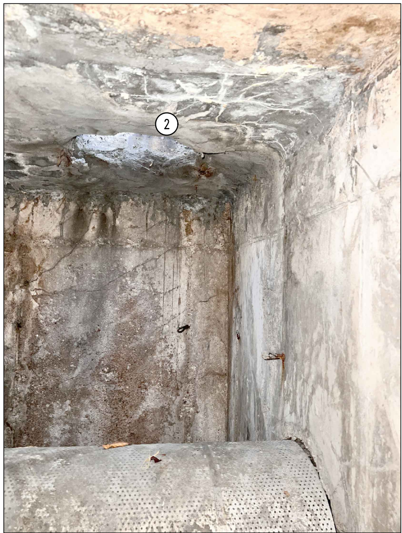
2 WIDESPREAD LID SPALLING. SEE NOTE #2.
