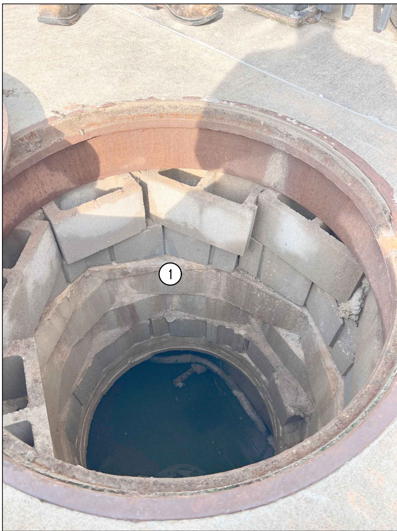
1 REMOVE PAVEMENT. REINSTALL CMU, THEN ADD REINFORCEMENT & GROUT INTO EXISTING HOLLOW CMU.
