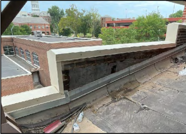
Figure (19) – ACM mastic along east parapet wall of c1920s Building.
