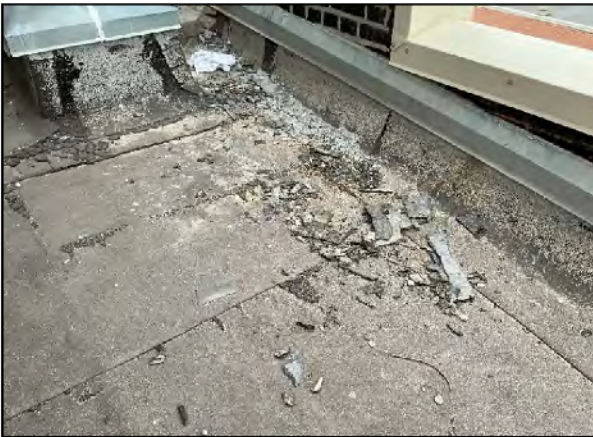
Figure (21) – ACM debris along Southeast parapet wall of c1920s Building.
