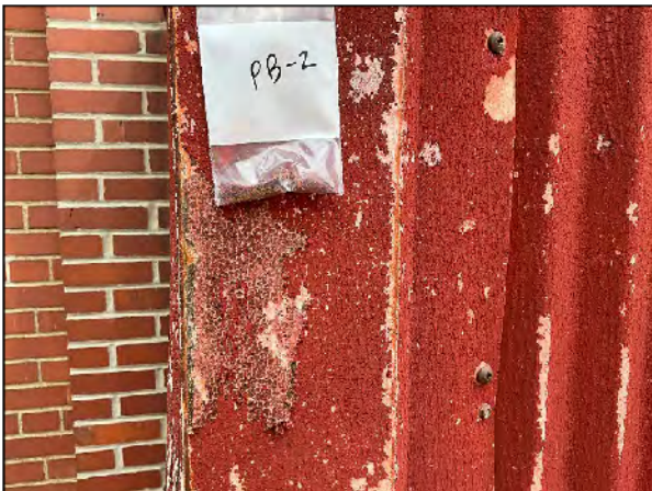
Figure (27) – Lead Bulk Sample PB-2 – Lead-Based Paint on Red Metal Siding.
