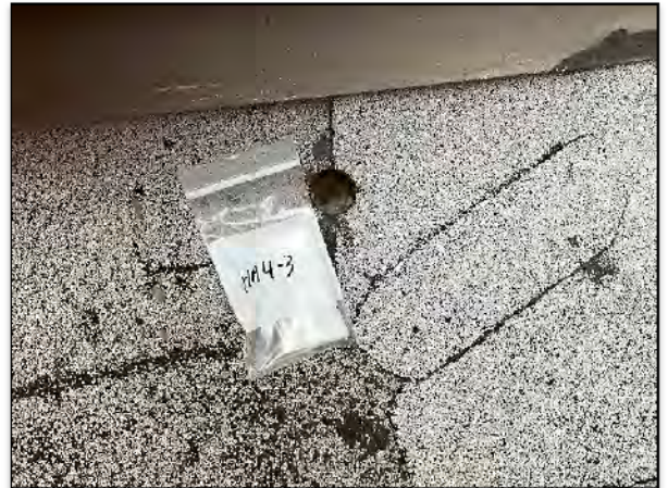
Figure (14) – Asbestos Bulk Sample HA4-3 – Flashing at Parapet Walls and Curbs.
