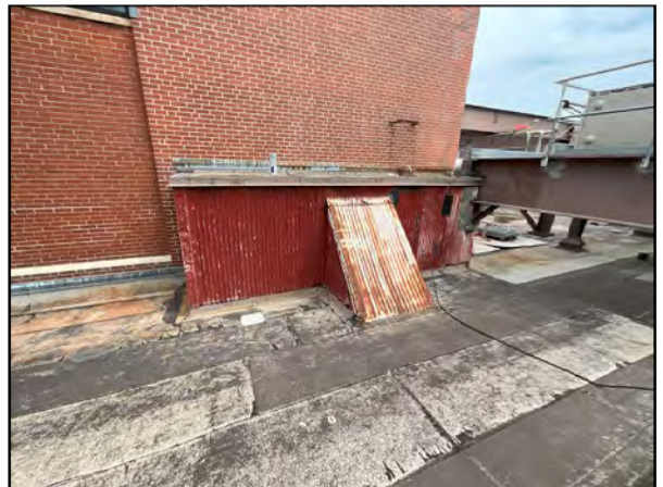
Figure (28) – Red Metal Shed with Lead-Based Paint.
