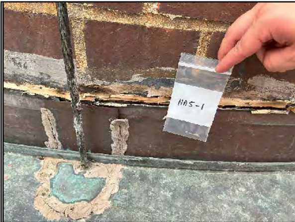
Figure (15) – Asbestos Bulk Sample HA5-1 – Tan Caulk at Brick Stack.
